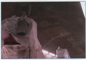
is ideal for vertical or overhead applications. Shotcrete MS is available in both dry-process and wet-process formulations.
