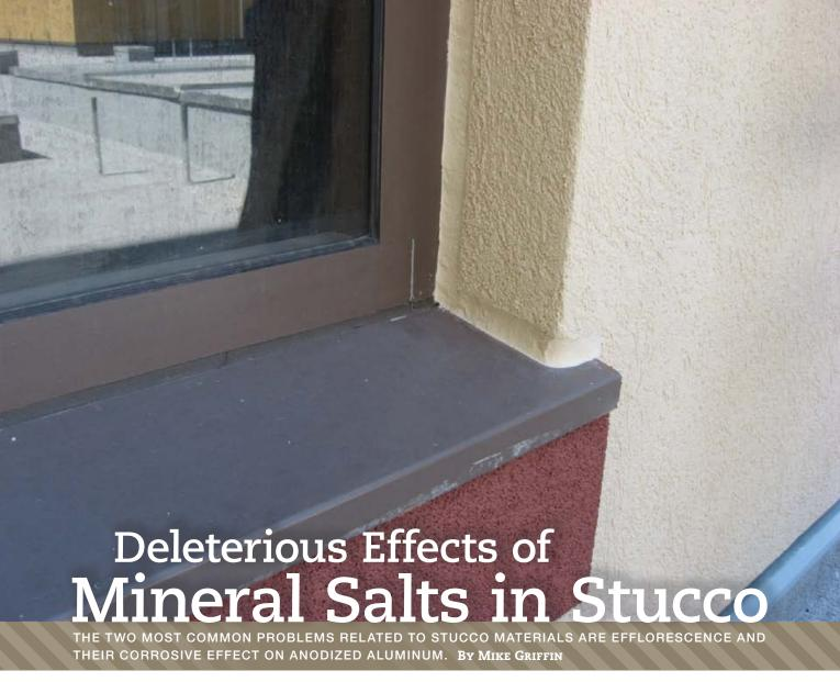
Efflorescence is the result of mineral salts deposited on the surface of stucco, EIFS, concrete or masonry. These deposits are typically harmless but can detract from the structure's aesthetics.
