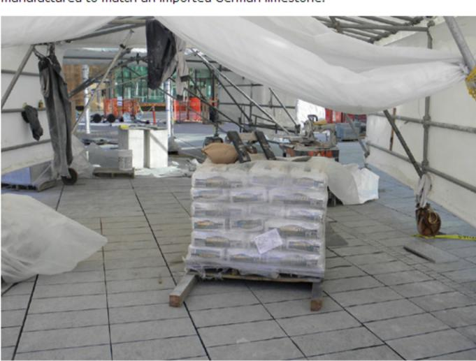
Quikrete Multi-Purpose Thin Set, a polymer modified thin set, was used for the installation of all interior stone tile. Quikrete Polymer Modified Veneer Stone Mortar exceeds the ASTM C 270 requirements for Type S Mortar and exhibits two-times the sheer bond strength of standard Type S Mortar.
