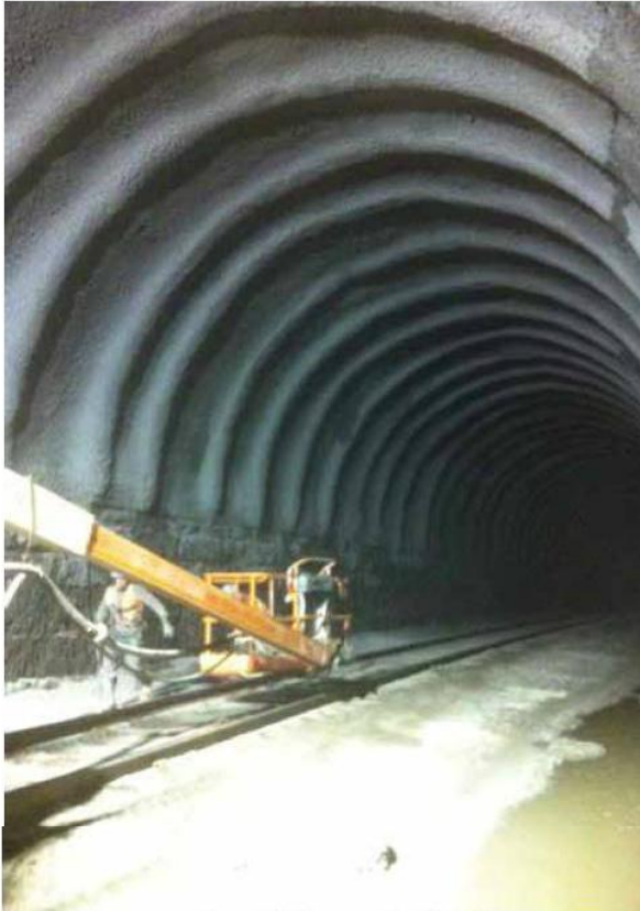
Fig. 4: Work was performed 24 hours a day for 28 days
