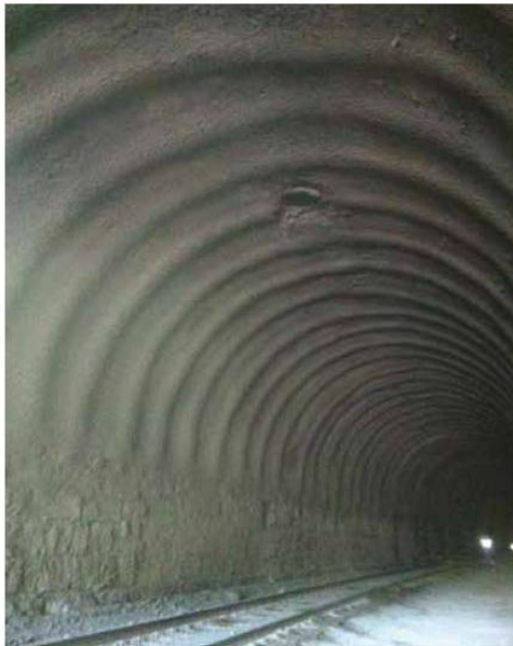
Fig. 1: Ribs 8 in. (203 mm) thick with 4 in. (102 mm) of shotcrete in between were placed
