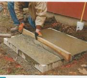
Screed the slab. Flatten the concrete using a straight 2x4 that's about 1 ft. longer than the form width. Move the board forward with a back-and-forth sawing motion while keeping it on the form.
