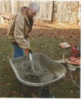
Mix the concrete. Dump two 80-lb. bags of mix in a wheelbarrow for each batch. Add 3 qt. of water per bag, and mix thoroughly with a hoe. Add small amounts of additional water if necessary to bring the concrete to a consistency that's about the same as thick cake batter.
