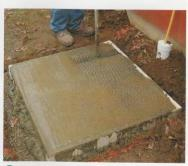
Tamp the surface with a rake. Gently tamp the entire surface of the slab. The rake pushes down the gravel that's part of the concrete mix, and brings up a mixture of cement and sand that's easier to smooth.
