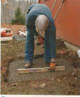
Qrade the gravel. Fill the excavation with 4 in. of gravel. Rake it flat, and use a level to make sure it's pitched about <sup>1</sup>/<sub>4</sub> in. per ft. so that the slab, which will parallel the base, drains water.
