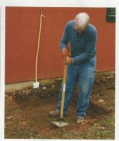
Prepare the subgrade. Dig 6 in. beyond where you want the slab edges and 8 in. deeper than where you want the top of the slab. Make sure the subgrade pitches away from the building, and tamp down loose soil.
