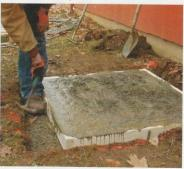
Tap the sides of the form. Lightly hammer the form all around the slab until you see bubbles rising from the concrete. This step makes for a smoother slab edge that won't collect water, which can freeze and spall the concrete.
