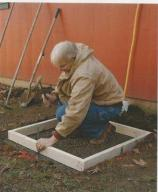
3 Make and set the form. Most 4-in. slabs are actually the 3½-in. depth of standard 2x4s. Nail the corners together, and place the form on the graded gravel, making sure it doesn't rock. Drive 12-in. lengths of rebar to just below the top of the form to keep it from moving.
