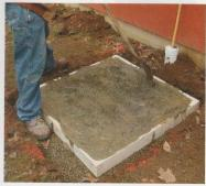
**5** Settle the concrete. After dumping the mixed concrete in the form, jab into it all along the edges with a shovel. This helps to ensure that the mix fills the form without leaving voids.
