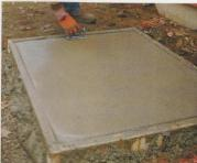
Round the corners. This leaves smooth, friendly edges that are less likely to chip. Use an edger once after each mag floating: on interior slabs with exposed edges, use it after the steel float. After the slab hardens for a day or more, pry the joints apart and remove the form.
