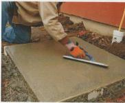
Smooth the rake marks with a mag float. Keep the leading edge of the float up. When the surface water dissipates, float the slab again. This is the final finish for exterior slabs. For a smooth interior slab, work it again with a steel float when the surface begins to lose its wet sheen.
