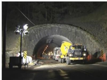
Shotcrete was applied up to 18 in. thick between existing timbers sets.
