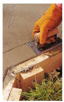
**10** Shape the edges of the concrete by running an edger along the forms. Smooth out any marks created by the edger using a float. Lift the leading edge of the edger and float slightly as you work.
