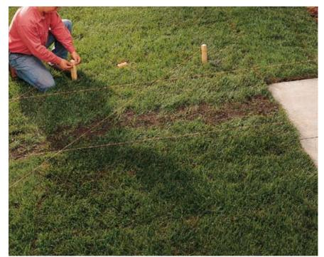
**Select a rough layout, including any turns.** Stake out the location and connect the stakes with mason's strings. Set the slope, if needed. Remove sod between and 6" beyond the lines, then excavate the site with a spade to a depth 4" greater than the thickness of the concrete walkway, following the slope lines to maintain consistent depth.
