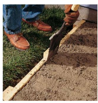
**7** After pouring all of the concrete, run a spade along the inside edges of the form, then rap the outside edges of the forms with a hammer to help settle the concrete.
