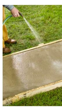
**13** Keep concrete damp by spraying periodically with a fine water mist or cover with plastic sheeting for five to seven days.
