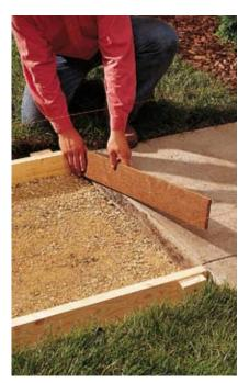
**4** Glue an isolation board to the steps, house foundation, or other permanent structures that adjoin the walkway using construction adhesive.
