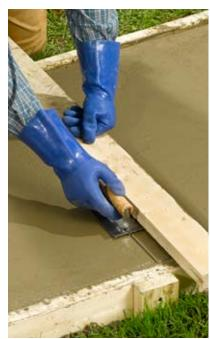
**11** Cut control joints in the concrete after the concrete sets up but before it hardens.
