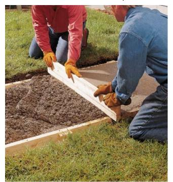
**8** Build a curved screed board and use it to form a crown when you smooth out the concrete. Note: A helper makes this easier.
