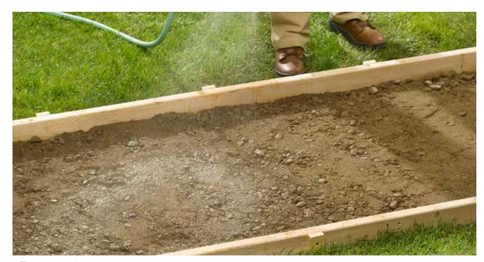
**5** Prior to placing concrete, it is necessary to dampen the gravel subbase. Spray the subbase using a water hose until saturated but do not leave standing water.
