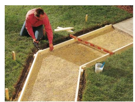
**3** Build and install 2 × 4 forms set on edge. Miter-cut the ends at angled joints. Position them so the inside edges are lined up with the strings. Attach the forms with 3" deck screws, then drive 2 × 4 stakes next to the forms at 3-ft. intervals. Attach the stakes to the forms with 2½" deck screws. Use a level to make sure forms are level or set to achieve the desired slope. Drive stakes at each side of angled joints.
