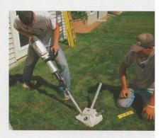
The residential models have a load capacity of 2700 lb. when installed in 1500-psf soil and 3600 lb. in 2000-psf soil. The pins are driven into the earth in just minutes using a 11/6-in. hex-shank demolition hammer.
