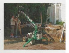
capacity of the footing. Once the required bearing is reached, the pile is cut to length and a beam saddle is welded on. Depending on the contractor, you can end up with an engineer's report that verifies the load each footing can handle. One source for that service is technometalpost.com.
