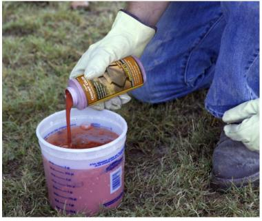
For a uniform mix, add liquid cement color to the mixing water, before mixing the concrete.
