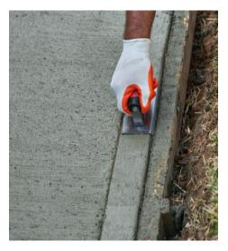
Finish and shape the concrete by making several passes with an edging tool.
