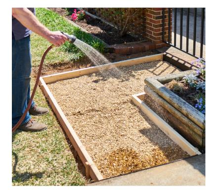
Proper placing and finishing techniques are essential to achieving a successful concrete project. Before placing concrete in the form, a properly compacted 4" gravel base should be dampened.
