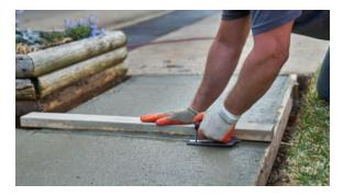
Use a groover and straight-edge to cut in control joints. Control joints are designed to allow for expansion, contraction and movement of the concrete slabs. 4" thick slabs require control joints a minimum of every 10 lineal feet. The control joint must be cut a minimum of 1/4 the depth of the slab.
