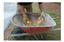
Hand mixing can be done in a mortar tub or wheelbarrow with a shovel or hoe.
