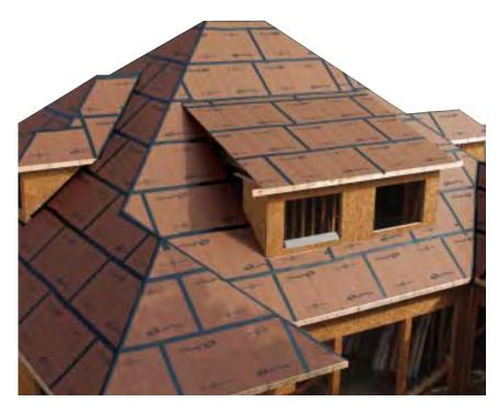
preventing water entry during roof-damaging storms, says Huber, the product protects the building's interior until the finished roofing is installed. The company also claims the Zip System is faster and easier to work with than felt and more durable as a temporary roof. Once labor costs are factored in, pricing purportedly runs about the same as for conventional OSB and felt.
