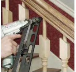
cost about \$3 apiece more than similarly styled conventional balusters, but because the system eliminates the need for a plowed handrail, the extra expense may be offset by savings of \$1.50 to \$3 per foot of rail.
