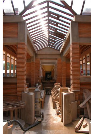
All told, King Bros. Masonry used 130 3,000-pound “super sacks” of QUIKRETE® Type N Mortar, formulated with white cement, Type S hydrated lime and aggregate from Frey Sand & Gravel, in addition to 120 “super sacks” of QUIKRETE® Type N Mortar, formulated with white cement, Type S hydrated lime and buff-colored masonry sand.
