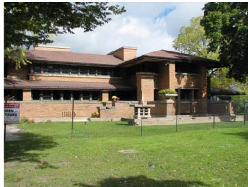
The project, the third in the four-stage restoration/rehabilitation plan, focused on rebuilding masonry walls, restoring face brick and matching mortar for the interior “backup” brick on the 10,000-square-foot main house, Martin House, and a 100-foot-long covered walkway (pergola) connecting the Martin House to an interior garden in the complex’s glass-roofed conservatory.
