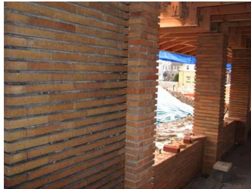
On the home’s exterior, there also were two different mortar colors used with the face brick; one color for the 5/8-inch thick bed joints, and another for the 1/8-inch wide head joints. This forced masons to use two separate trowels and mortar boards to keep the mixes separated.
