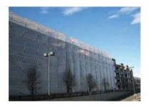
cycles if a driving rain hits it and it freezes. Cold conditions, as such, can also make the wall more susceptible to efflorescence forming on the surface of the wall. To counteract these cold weather problems several precautionary measures can be taken which may involve enclosing and heating the structure.
