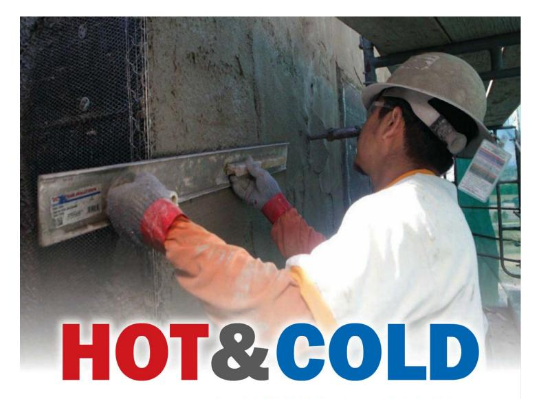
Weather has a significant effect on the application requirements and nuances of plaster/stucco seasonally, and sometimes daily. Contributing factors are: temperature, humidity, wind and the exposure of the sun.
