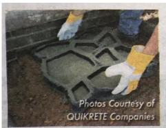
**Step 3:** Lay form at the beginning of the path and fill with concrete mix; smooth surface with a trowel.
