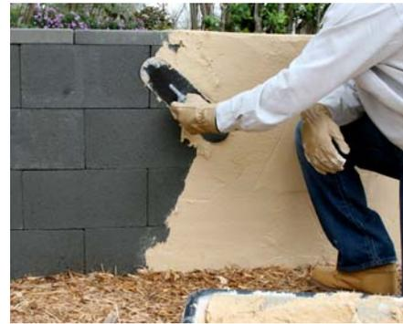
The material is code approved for mortarless wall construction, providing the construction design otherwise meets code requirements. The one-coat application provides structural strength and a textured “stucco” finish, in addition to sound-control and waterproofing properties.
