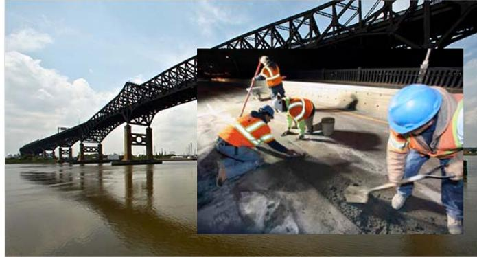
Because the 3.5-mile-long elevated structure is such a heavily-traveled thoroughfare, carrying more than 67,000 vehicles every day, the bridge must remain open for commuter traffic, especially during rush hours. That means crews can only close the road at night to make the much-needed repairs.
